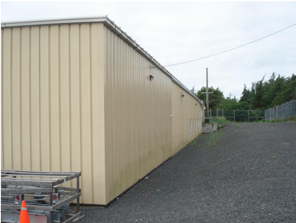
Photo 6 - Rear of Main Building
