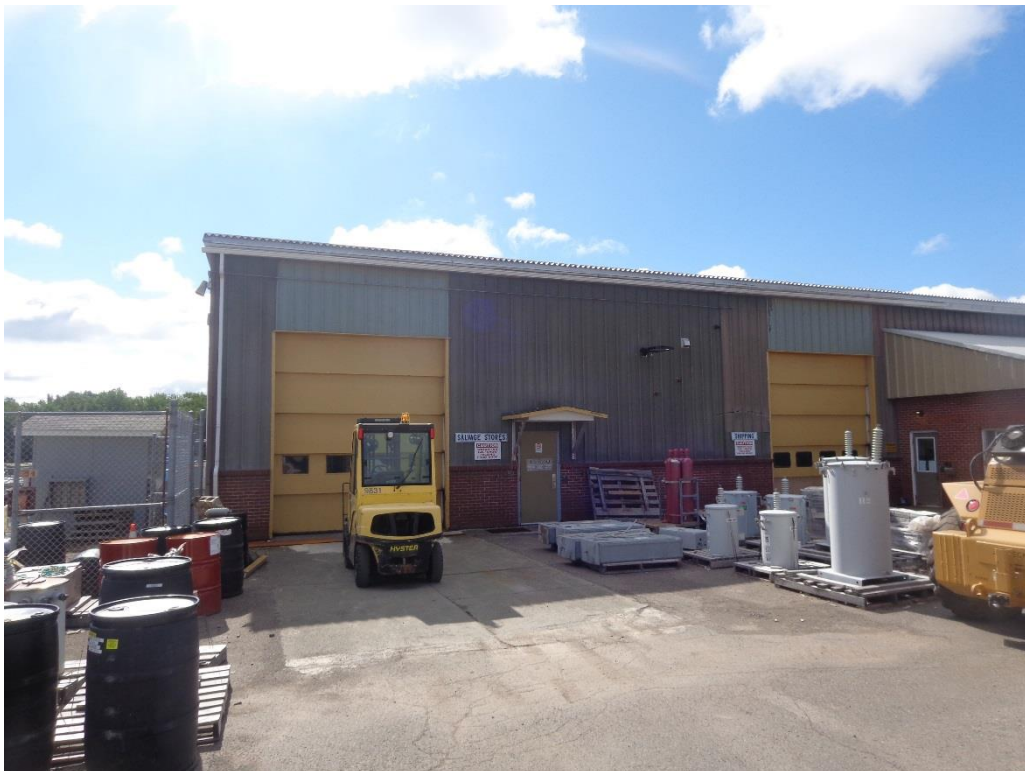
Photo 18 - Brick Veneer and Metal Cladding
