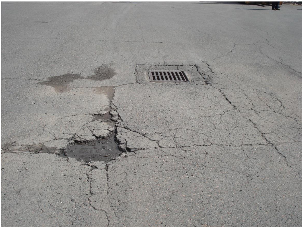
Photo 2 - Asphalt Degrading
