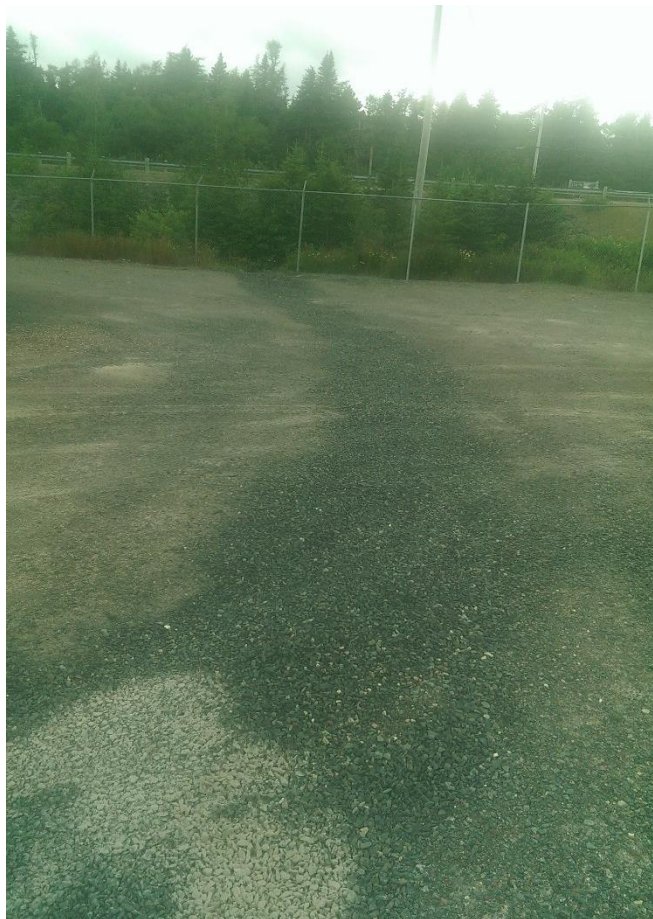
Photo 8 - Path of Storm Drainage
