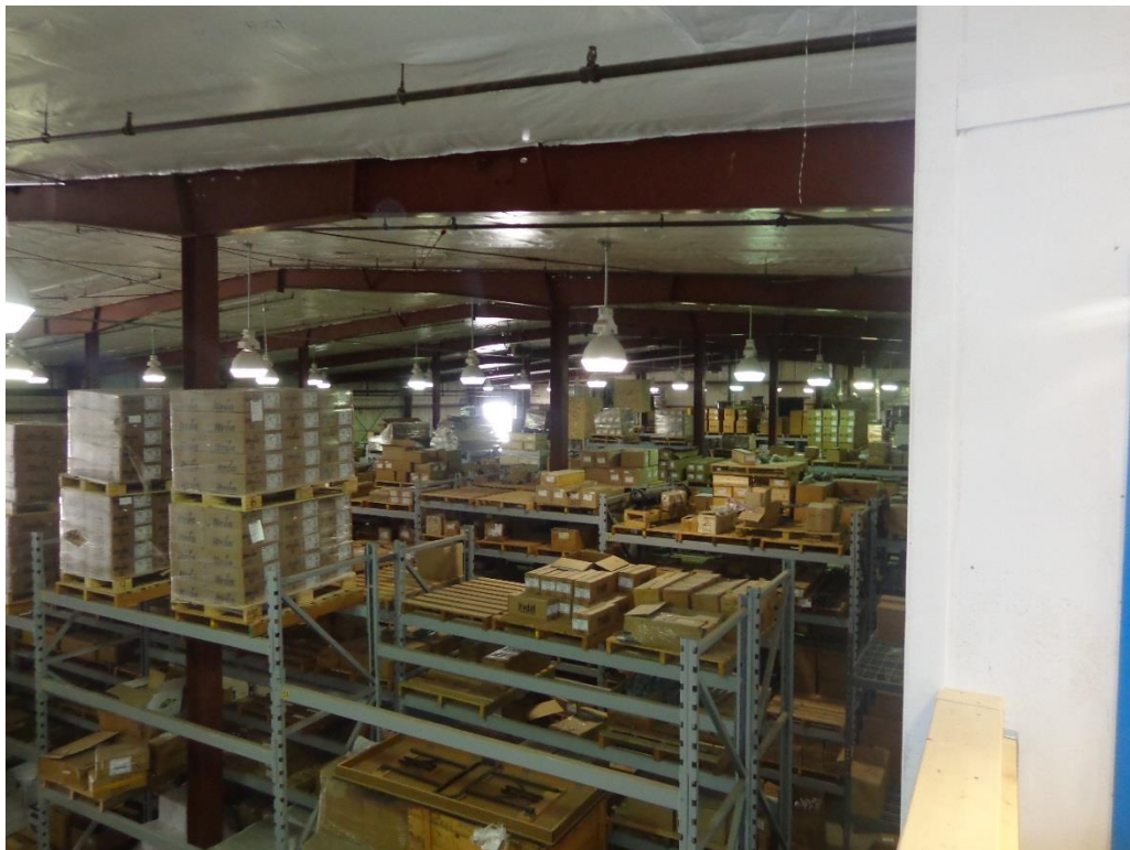
Photo 8 - Typical Building Frame
