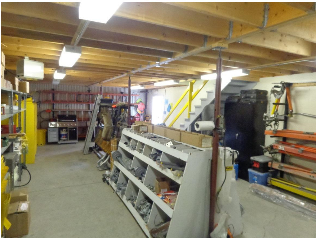
Photo 10 - Second Level Floor Framing
