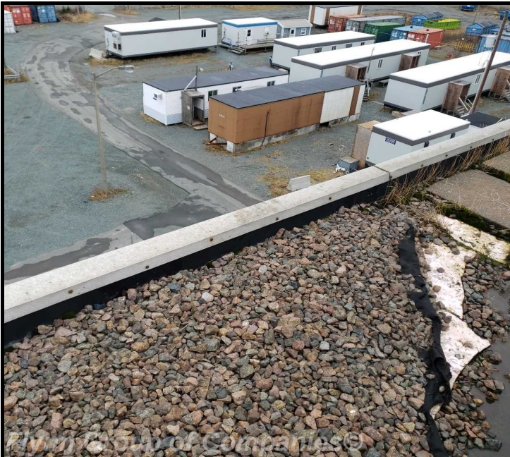
pump house #2: Fasteners
