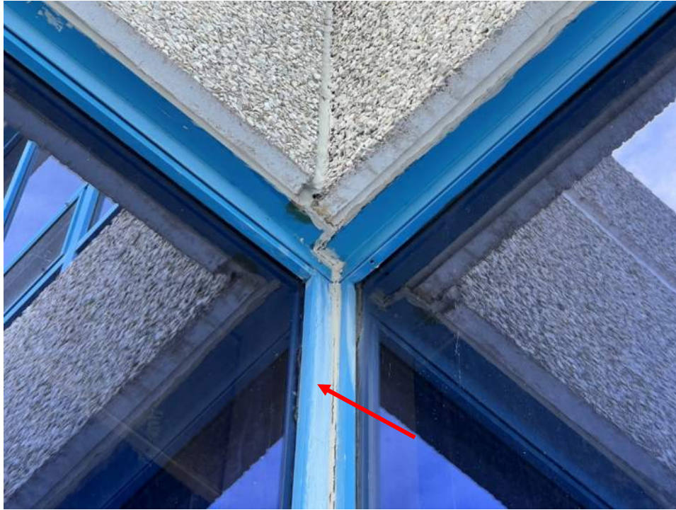
Photo No. 27: Typical view of adhesive sealant (red arrow)
