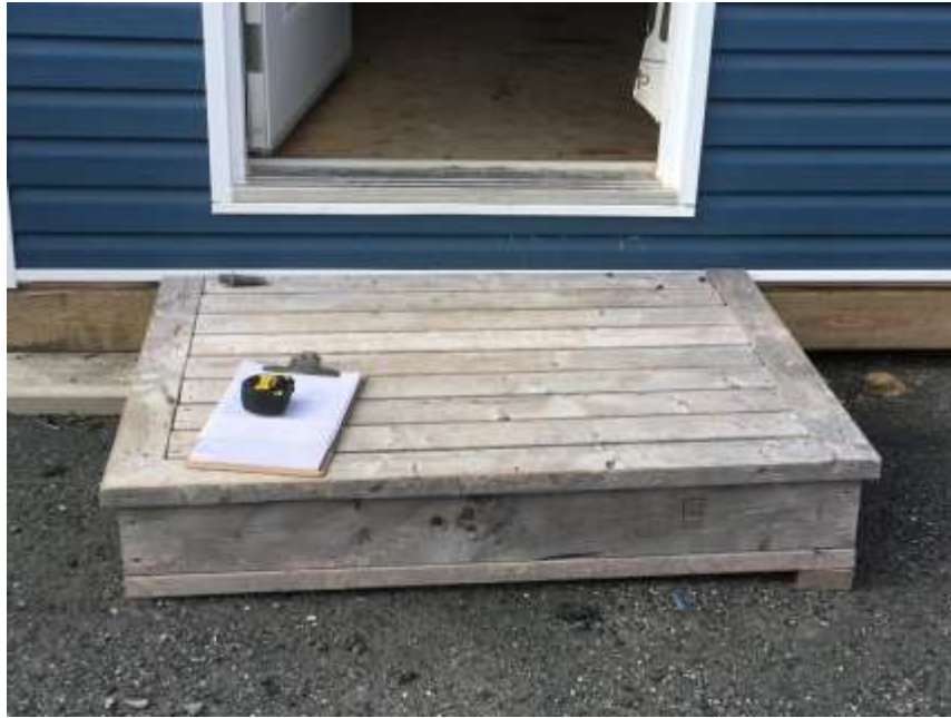
Entrance - note risers height.
