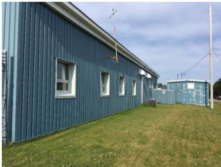
Rear façade with lean-to and storage building in background.
