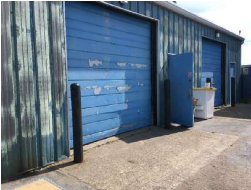
Partial front façade.
