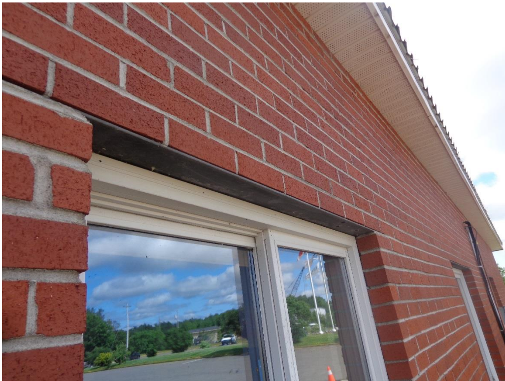
Photo 20 - Steel Lintel Over Window Openings
