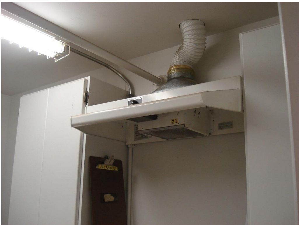
Photo 40 - Oil Test Lab Exhaust Hood
