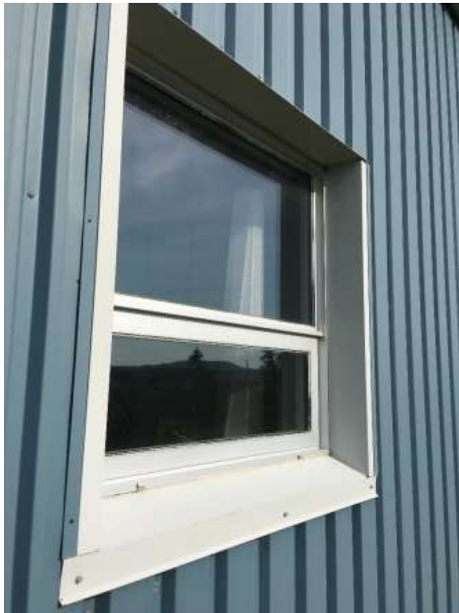
Typical window. Note deep reveal indicating added insulation and cladding.
