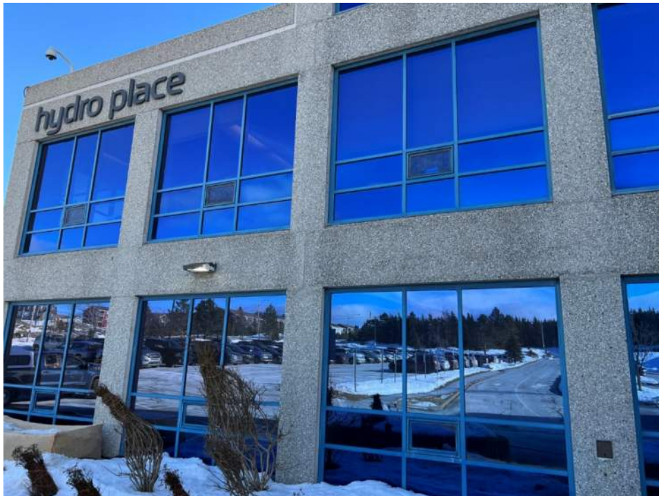
Photo No. 4: Overview of the west elevation
