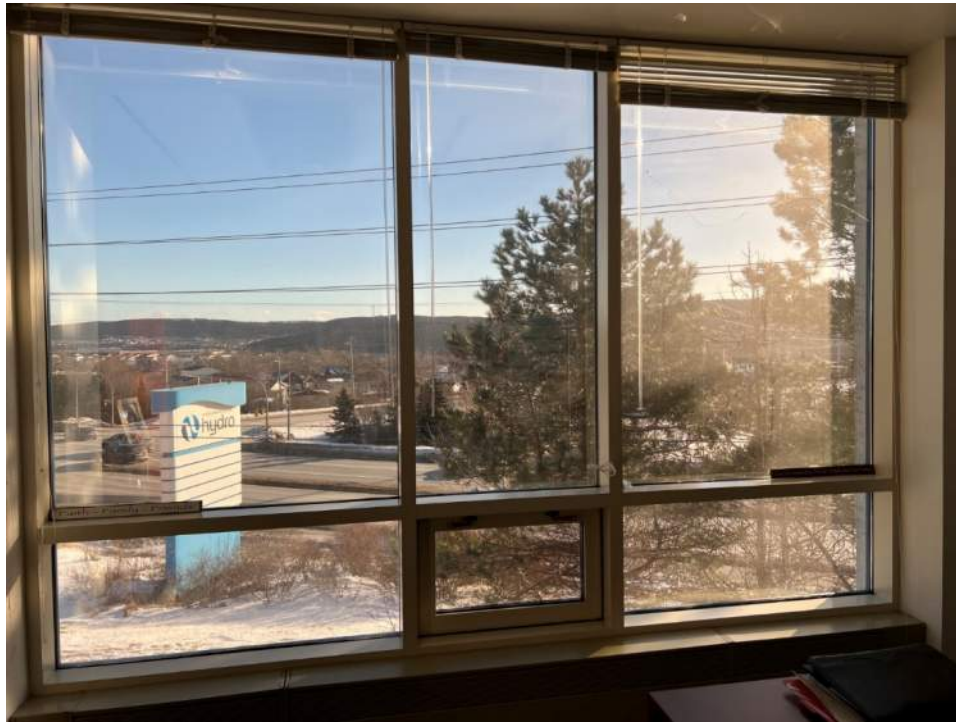
Photo No. 9: Overview of curtain wall is in fair-to-poor condition overall
