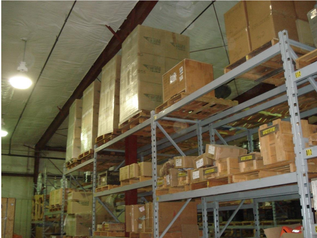
Photo 47 - Rack Storage Very Close to Roof
