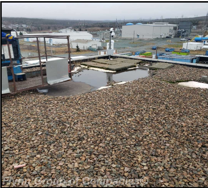
pump house #2: View of wind damaged area
