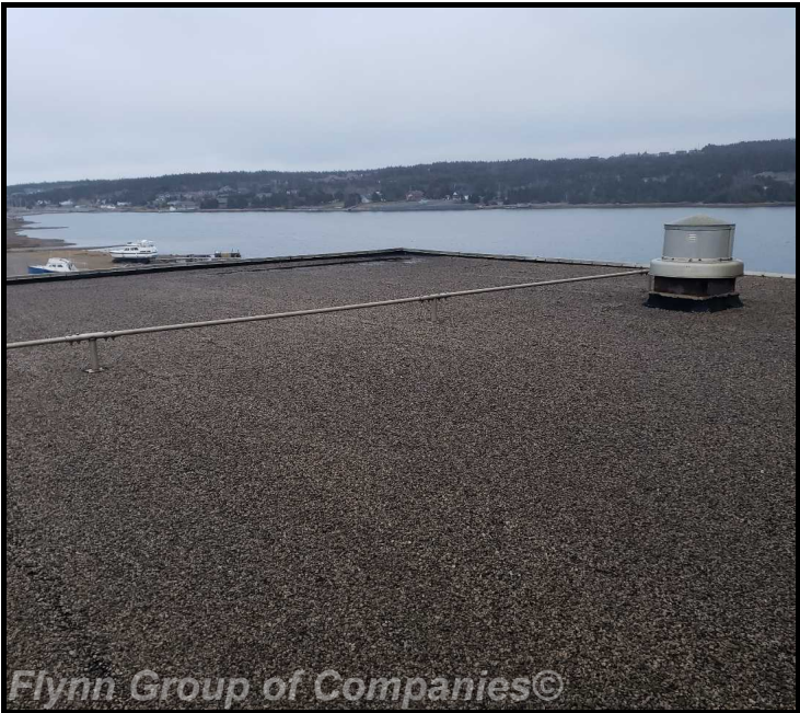
pump house #1: Overview of roof area
