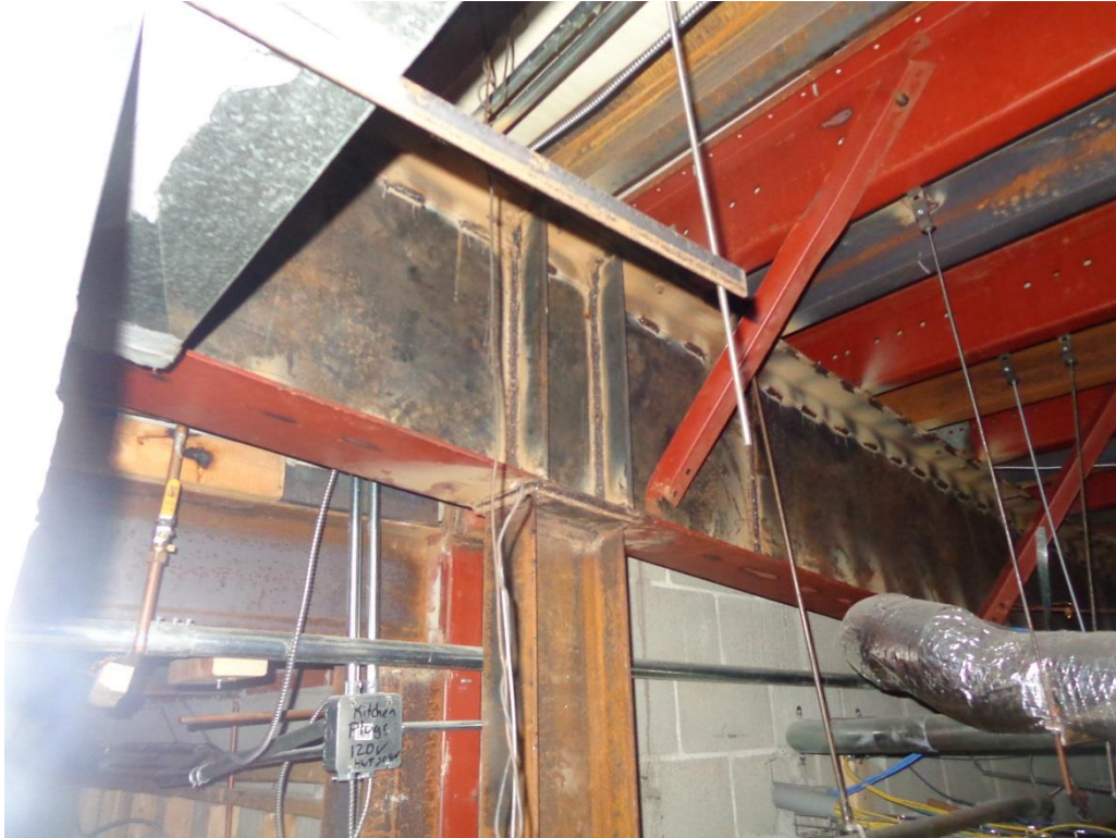
Photo 5 - Reinforced Building Frame
