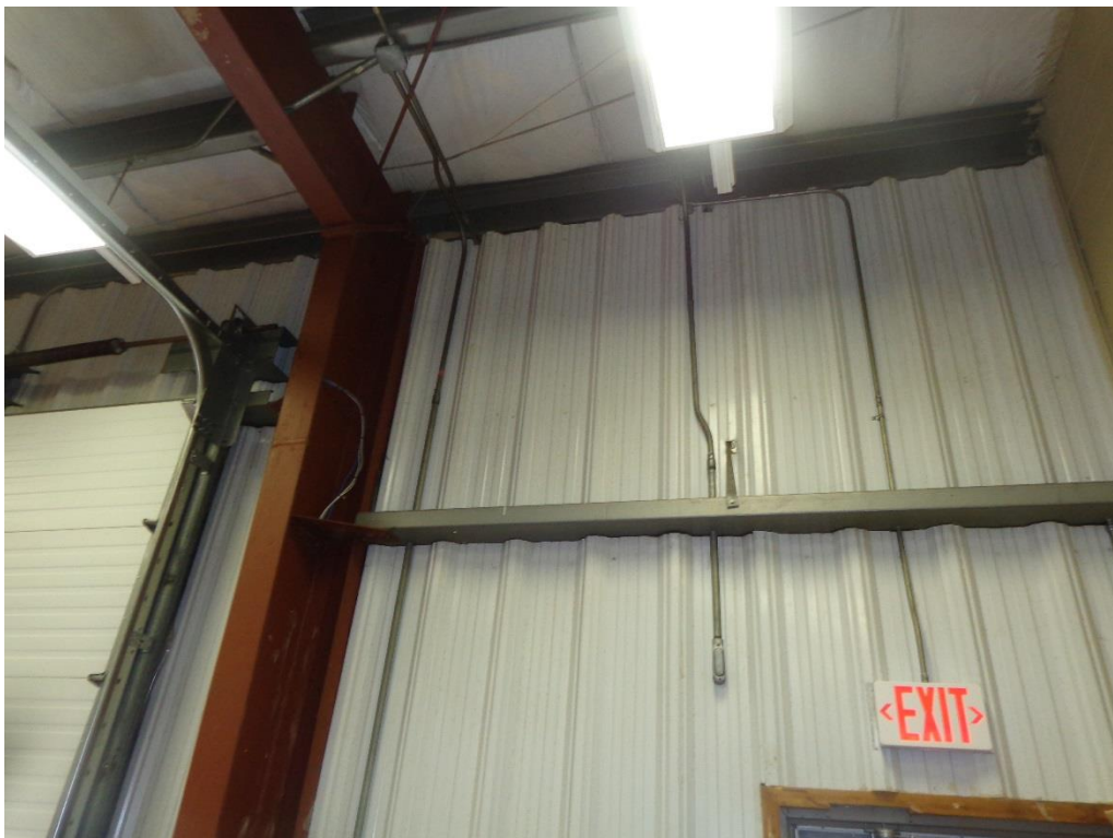
Photo 8 - Wind Girt Spacing and Paneling
