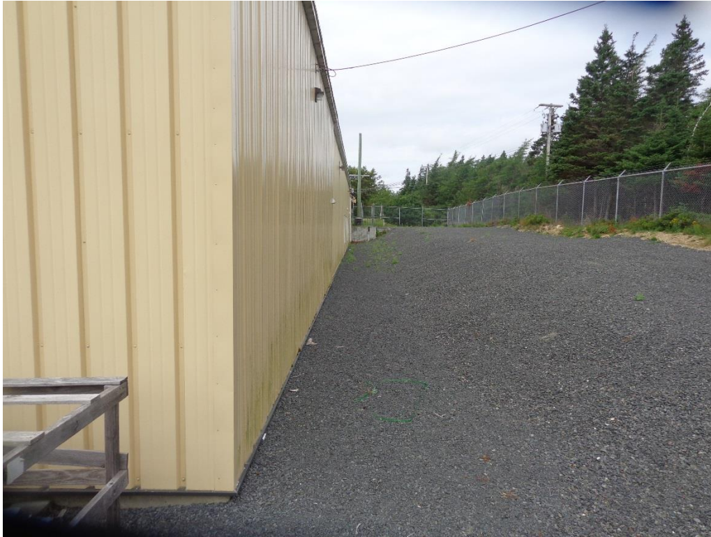
Photo 1 - Site Grading Towards Foundation Wall
