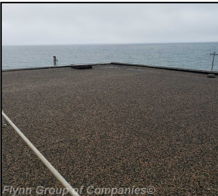
pump house #1: Overview of roof area - clean of debris
