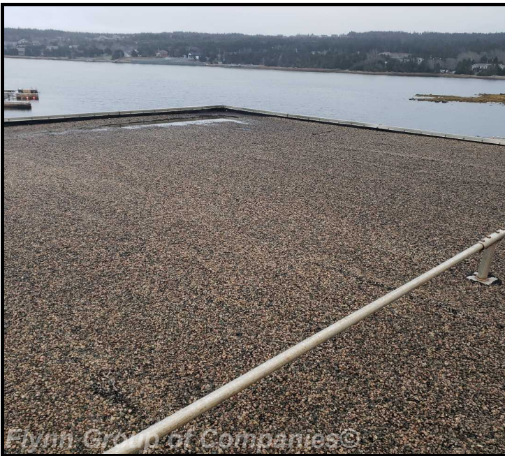
pump house #1: Overview of roof surfacing
