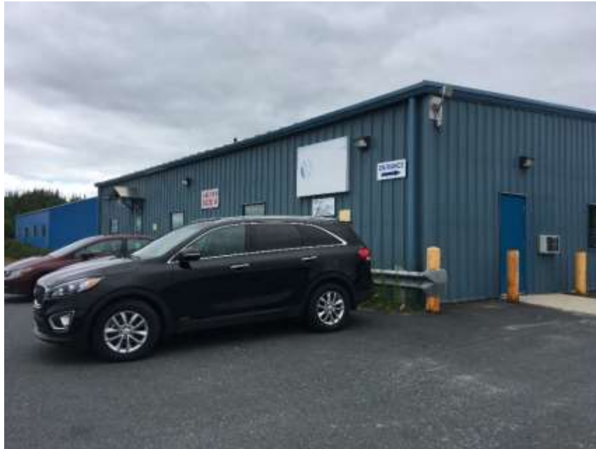
Front facade and partial right.
