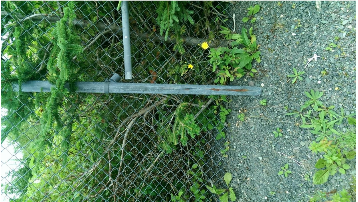
Photo 13 Pole Split and Brace Off
