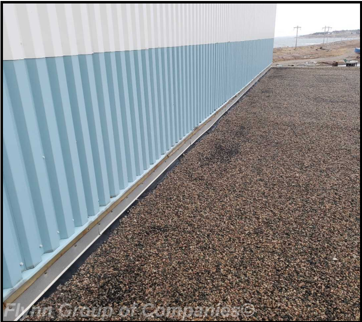
pump house #1: Area of lower roof level walls in good condition
