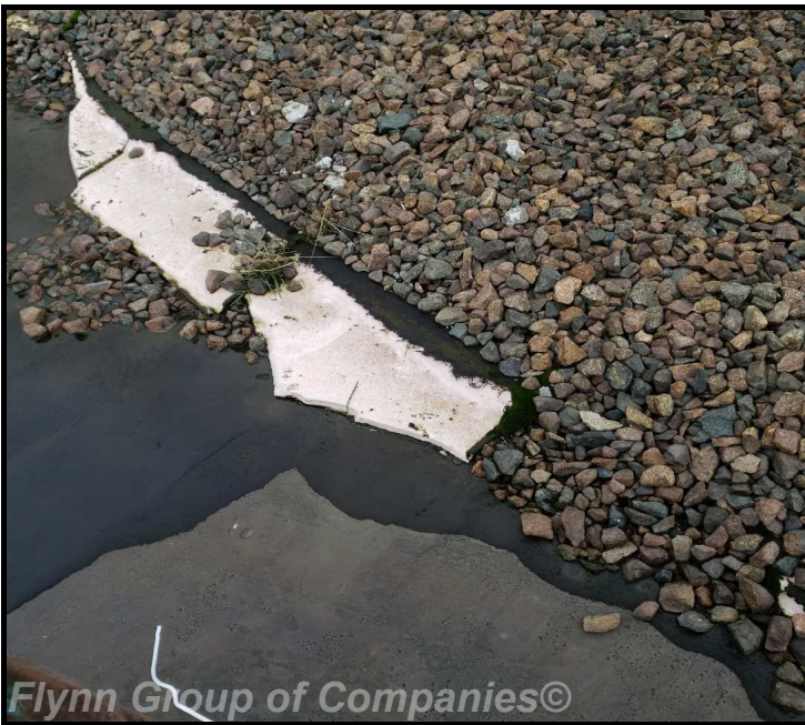
pump house #2: Roof composite
