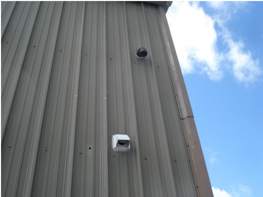
Photo 4 - Vent Piping Terminating Through Exterior Wall
