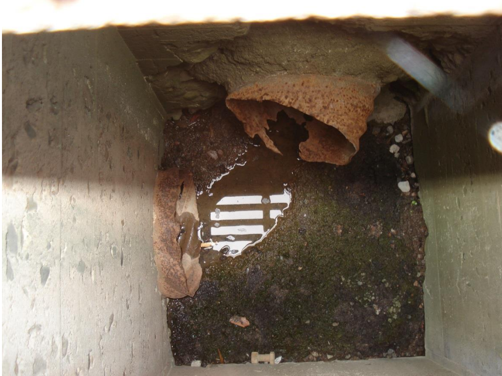
Photo 13 - CMP Corroded
