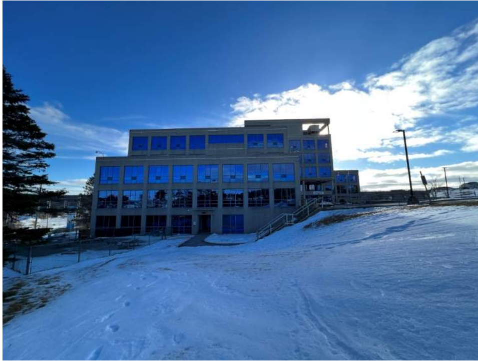
Photo No. 3: Overview of the south elevation
