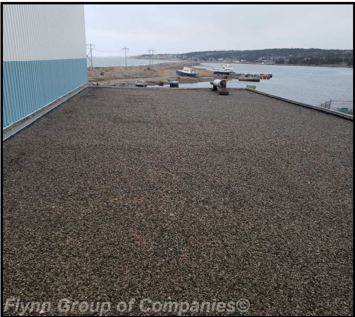
pump house #1: Overview of roof area - in good condition
