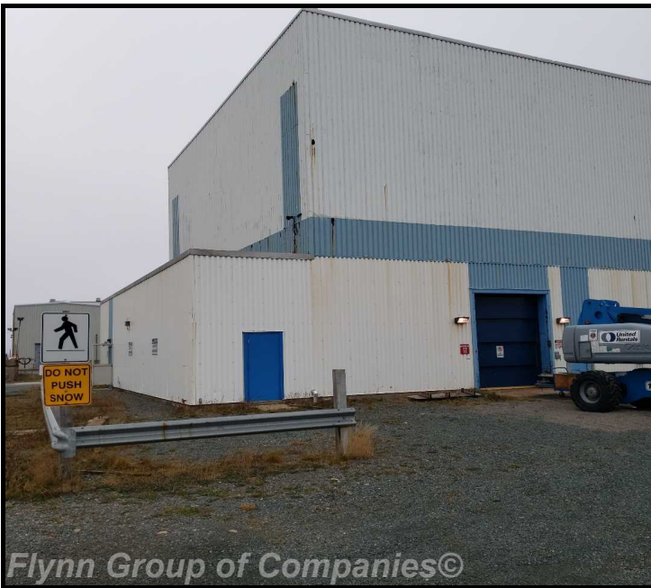
Front of Building: View of pump house #2
