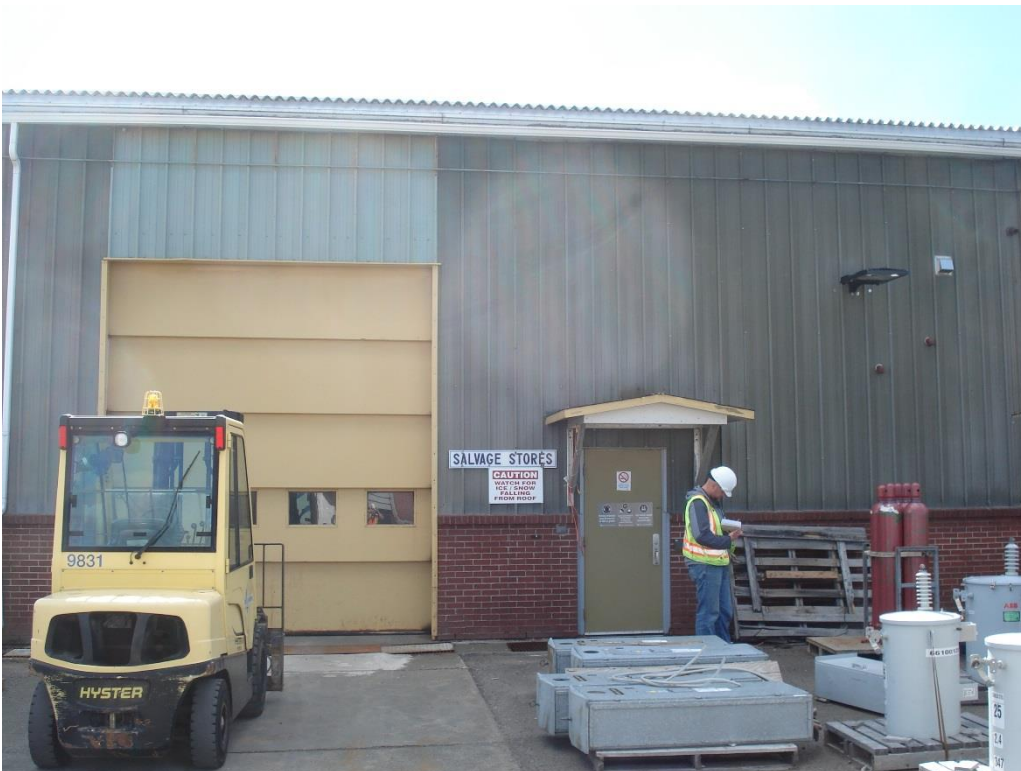
Photo 6 - Concrete Pad at Loading Door
