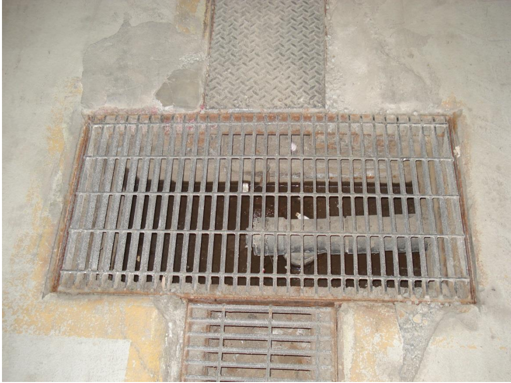
Photo 5 - Truck Bay Trench Drain
