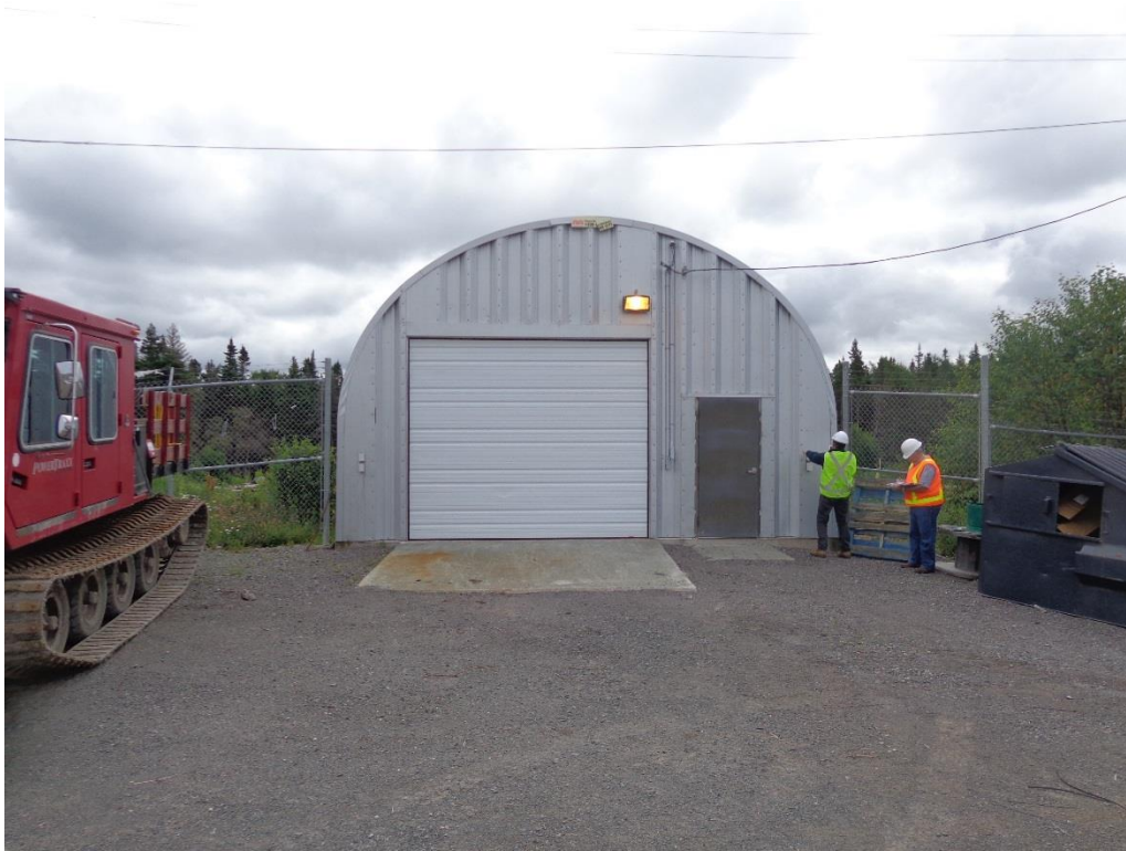
Photo 1 - Quonset Hut Structure
