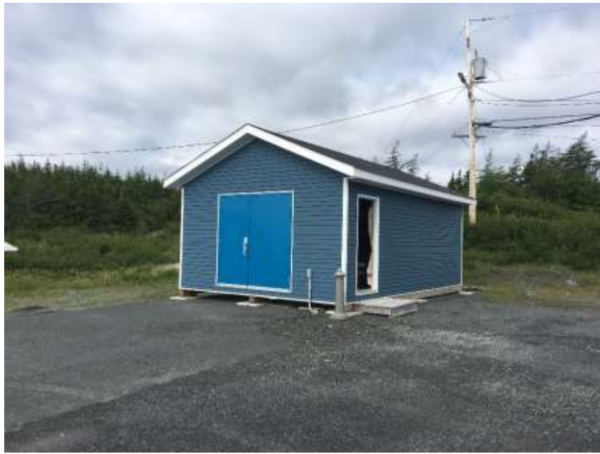
Front façade. Right side façade.
