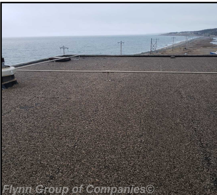
pump house #1: Overview of roof area
