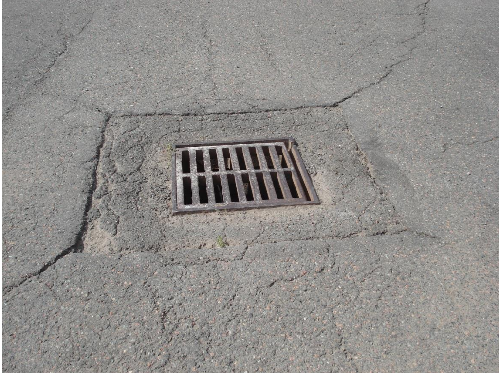
Photo 9 - Stormwater Catch Basin
