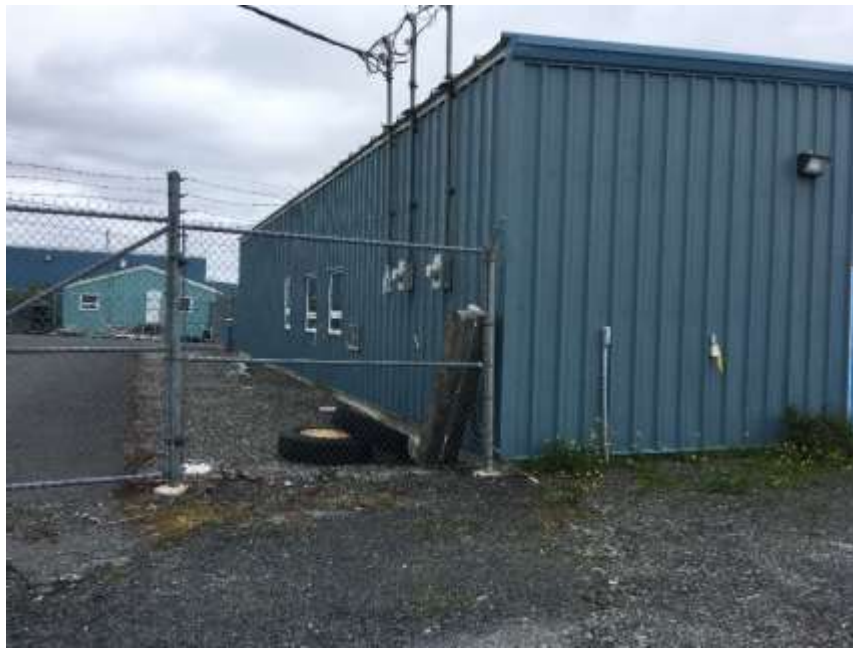
Rear façade and partial left.
