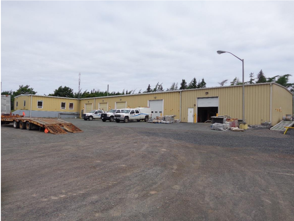
Photo 3 - Yard South of Main Building
