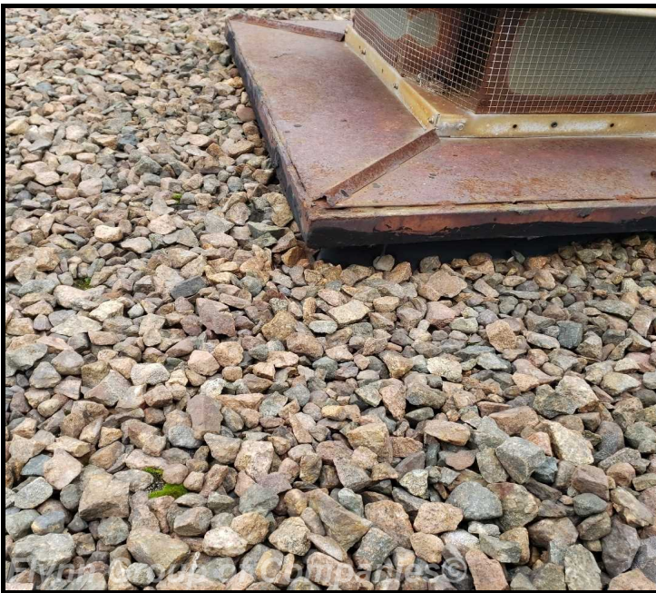
pump house #2: Curd detail flashing
