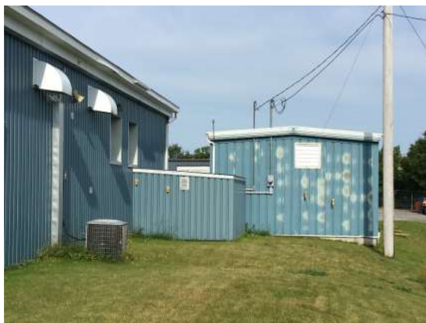
Partial rear façade with lean-to and storage building in background.
