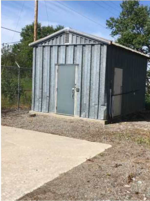
Exterior front and right facades.
