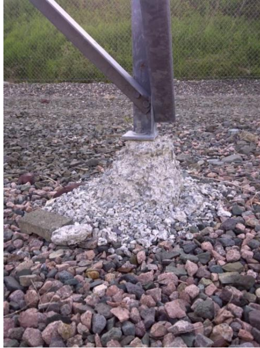
Figure 15: Structure L01L37-1 Western Avalon Terminal Station
