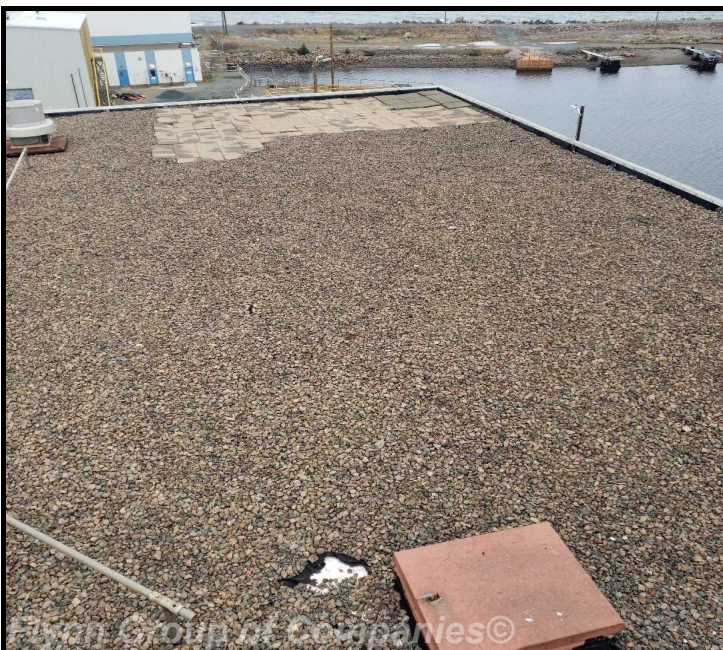
pump house #2: Overview of roof area
