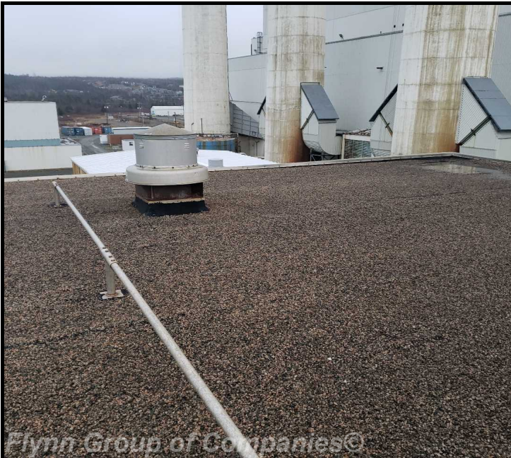
pump house #1: View overall condition of roof in good condition
