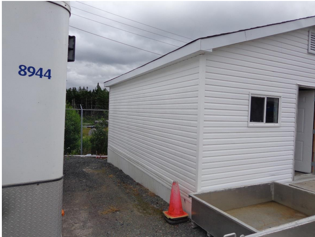
Photo 1 - Skirting Along Bottom of Building
