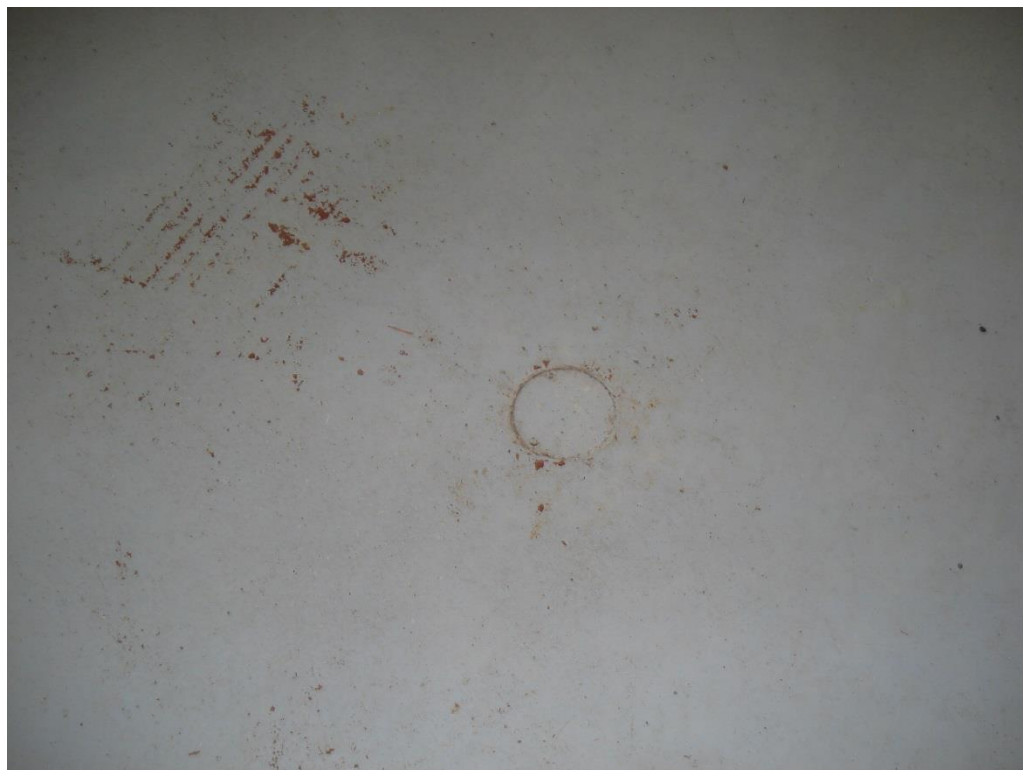
Photo 4 - Capped Floor Drain
