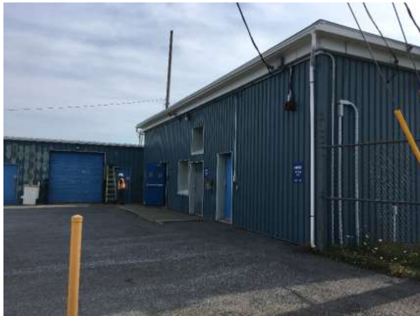
Main building shops access with storage building in background.
