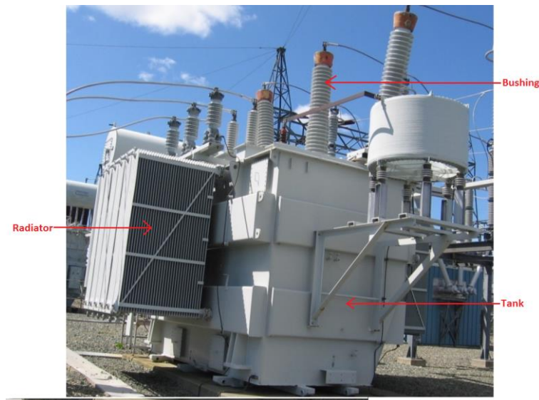
Figure 8: Power Transformer
