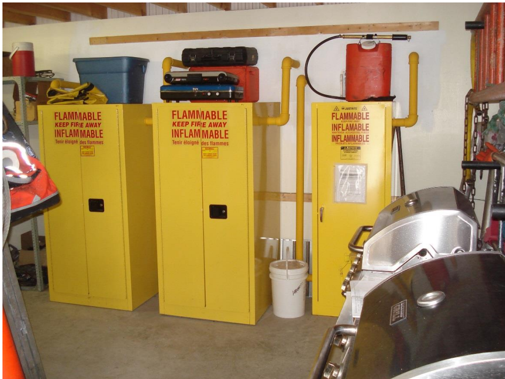
Photo 8 - Warehouse Extension Safety Cabinets
