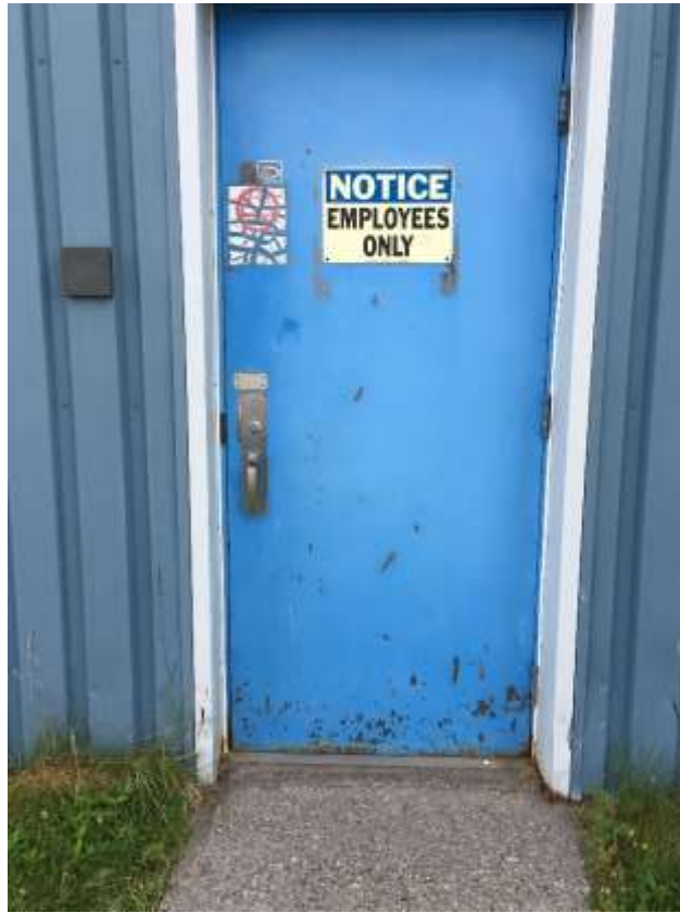
Representative exterior door.
