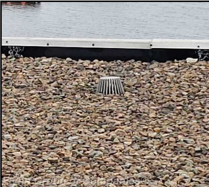
pump house #2: Drains clear of debris
