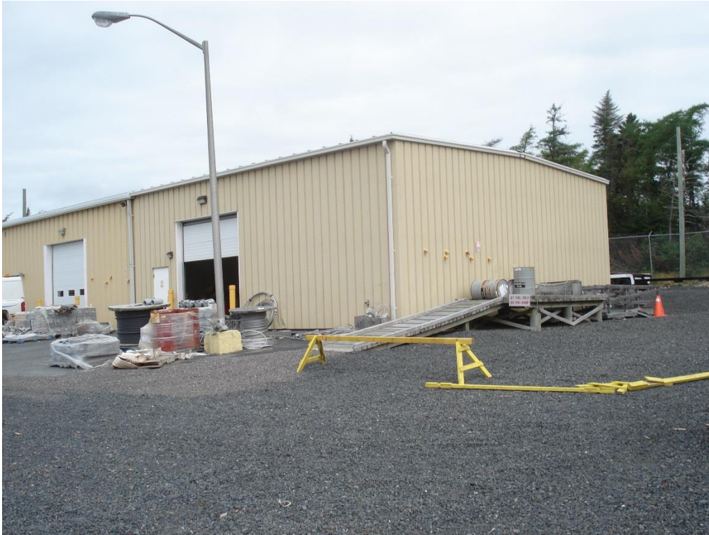
Photo 5 - East End of Main Building
