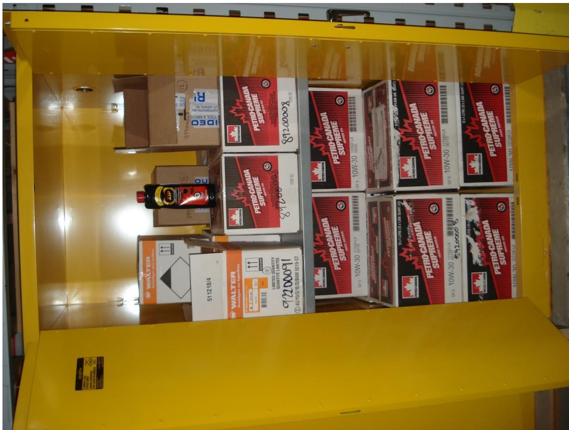
Photo 1 – Warehouse Safety Cabinet
