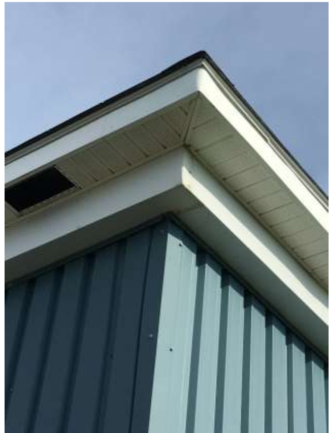
Typical roof soffit/fascia. Note double roof.
