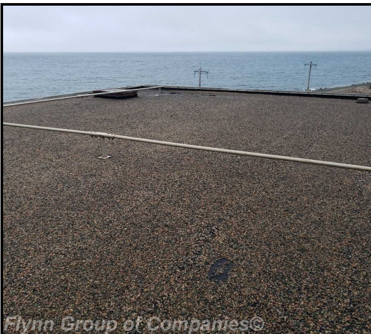
pump house #1: Area of roof 4 ply tremco rubberized and gravel
