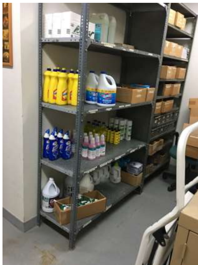
Janitorial supplies, which require rated room enclosure.
