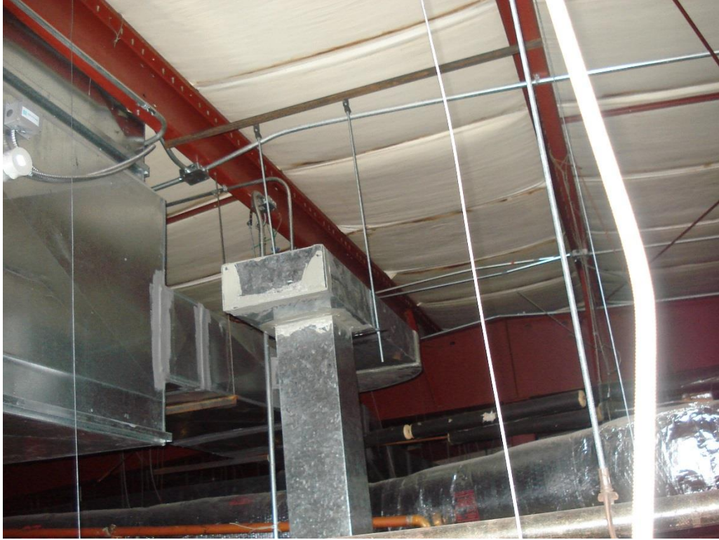
Photo 7 - Partially Insulated Domestic Water Piping
