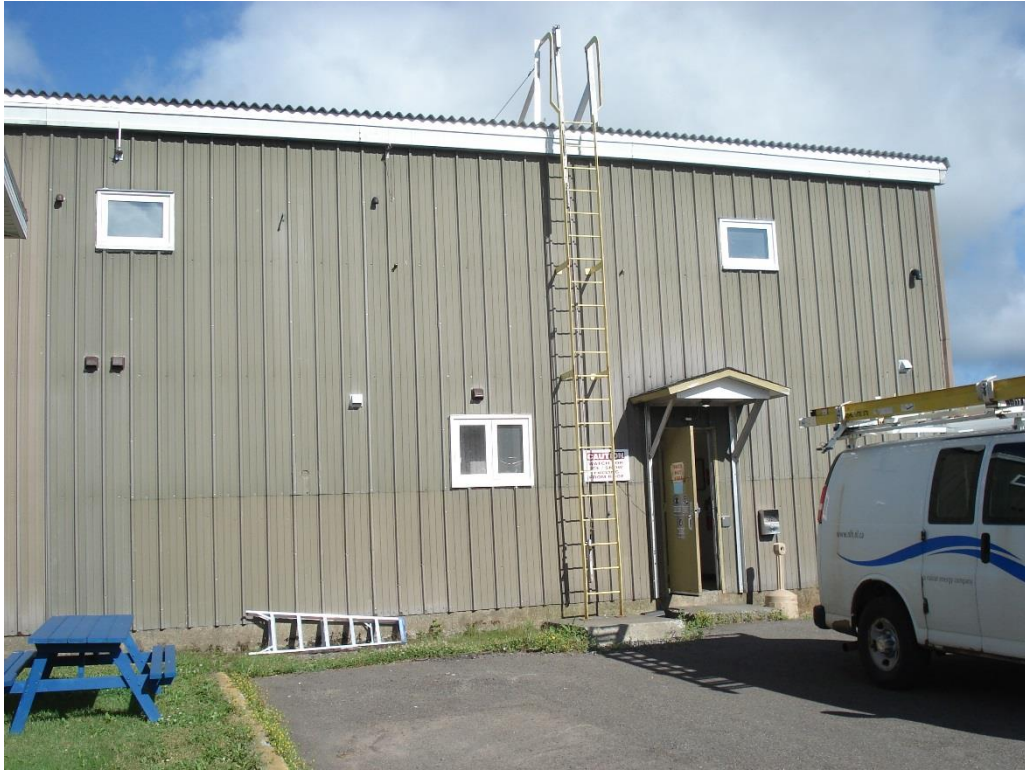
Photo 7 - Doorway and Equipment
