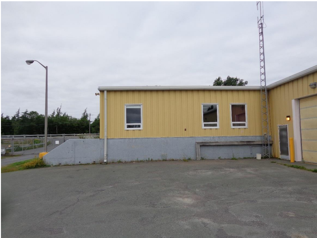
Photo 4 - Office Leg of Building
