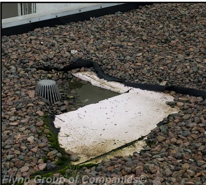
pump house #2: View of exposed insulation
