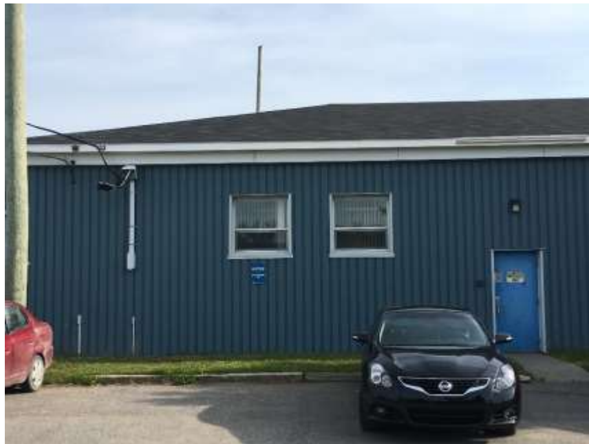
Hip roof above original roof.
