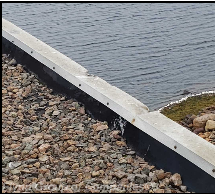
pump house #2: Areas of damaged metal
