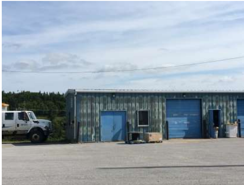
Partial front façade.
