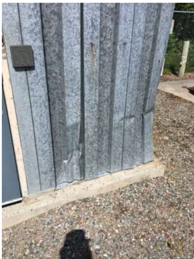
Cladding damage.
