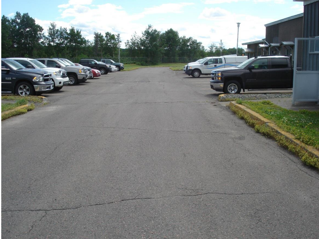
Photo 1 - Asphalt Cracking
