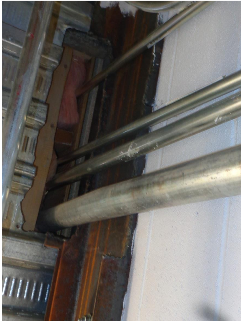
Photo 15 - Channel's Flanges Removed
