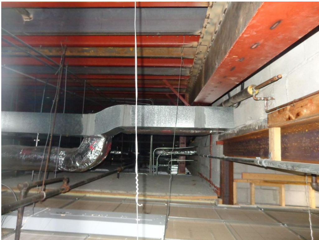
Photo 6 - Reinforced Building Frame and Additional Purlins
