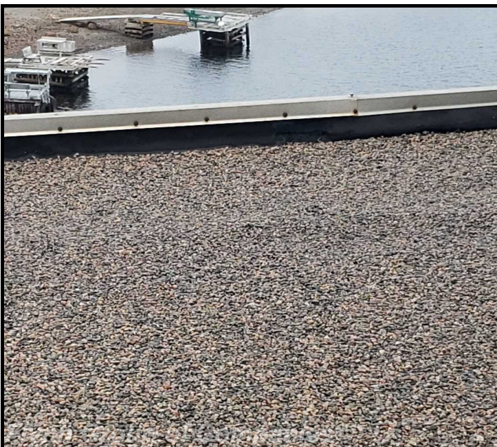
pump house #1: View of fasteners in good condition
