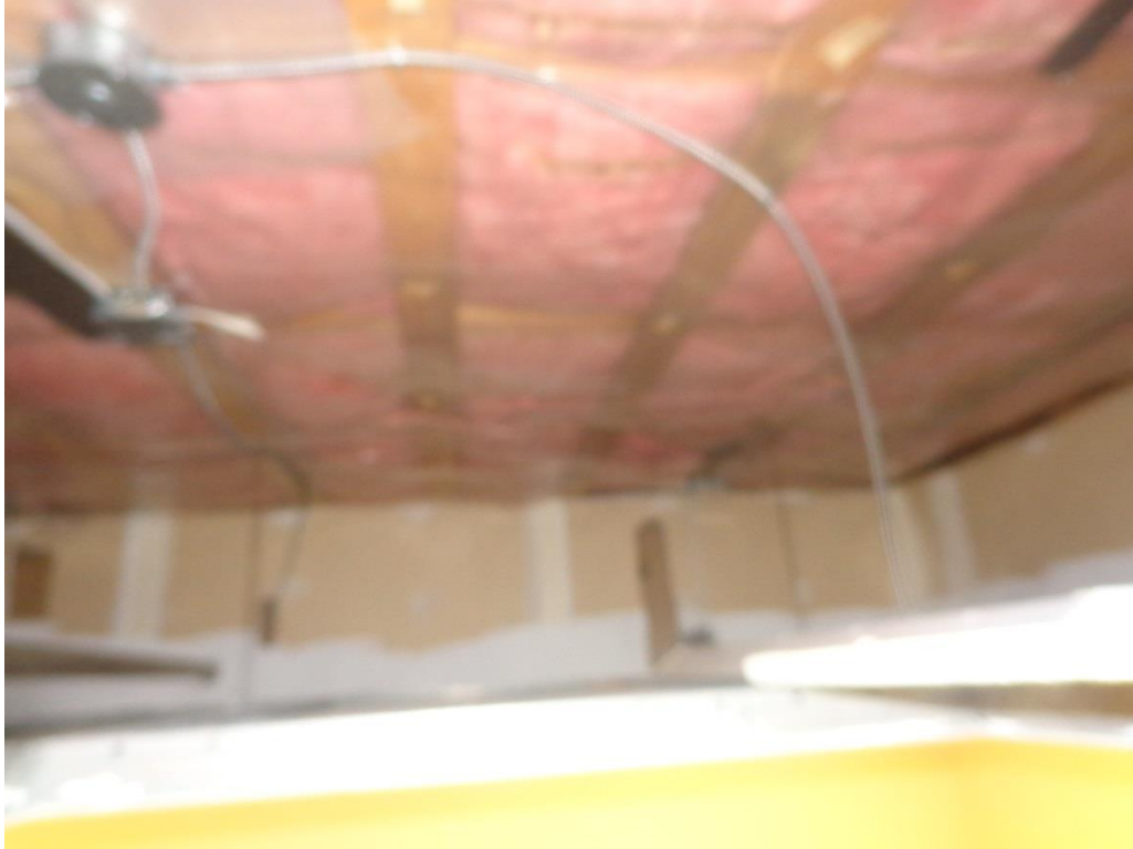
Photo 7 - Timber Trusses Concealed by Vapor Barrier and Insulation
