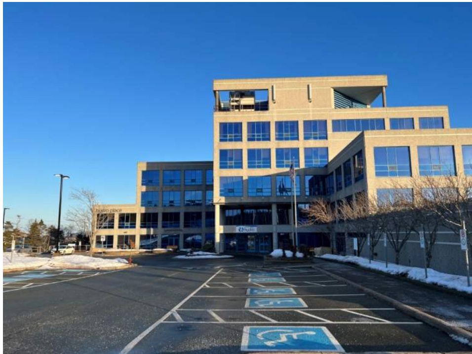
Photo No. 2: Overview of the west elevation
