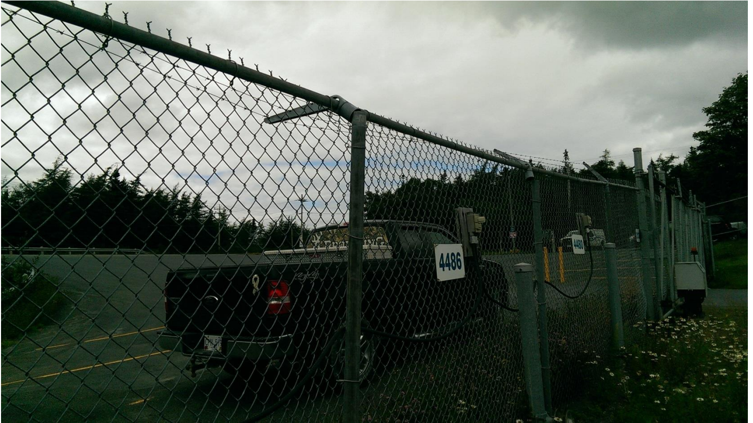
Photo 19 - Barbed Wire Supports Off
