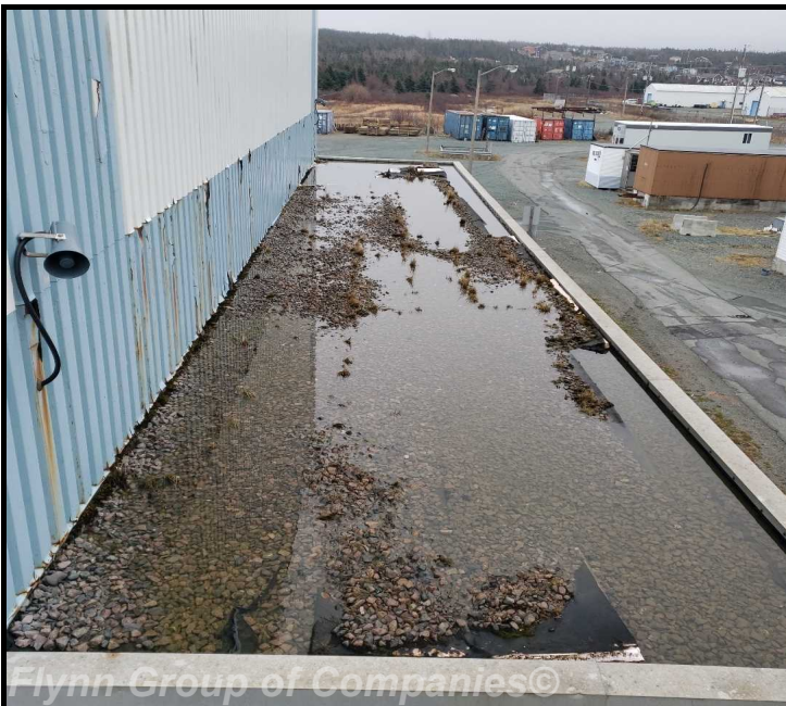
pump house #2: View of area of roof on pump house #2 at lower roof drain plugged and wind damage to roofing
